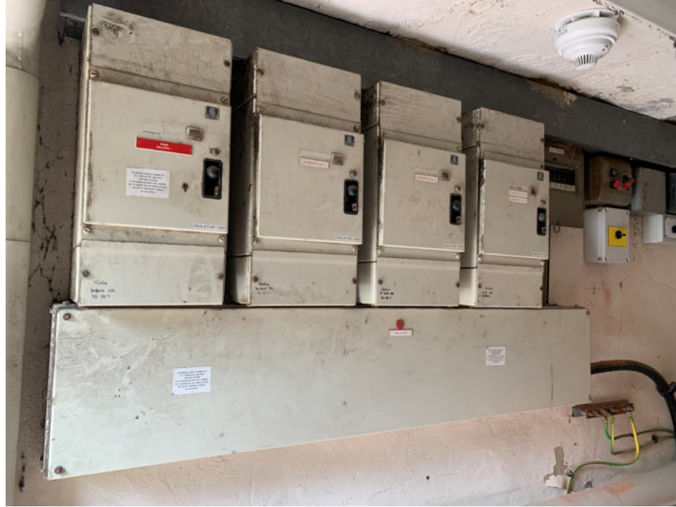
North Block Main LV Switch Panel
