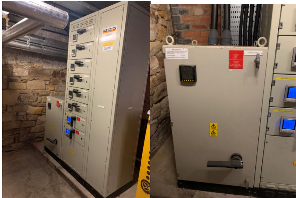
North Block Main LV Switch Panel
